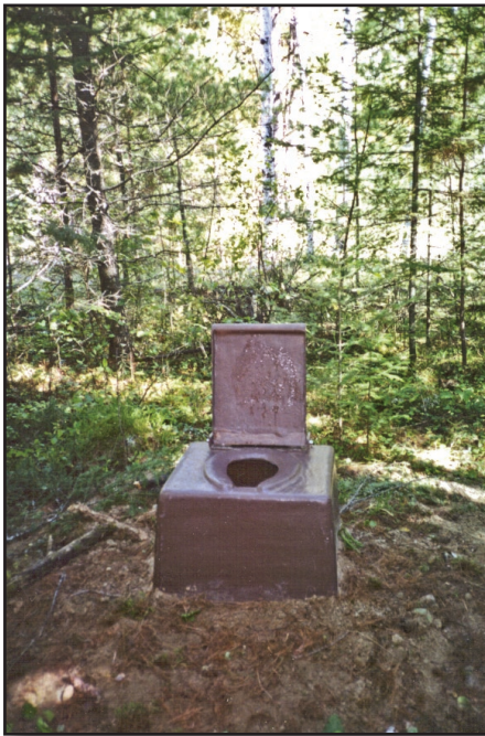
Figure 109—A fiberglass riser for a pit toilet in the Boundary Waters Canoe Area.
