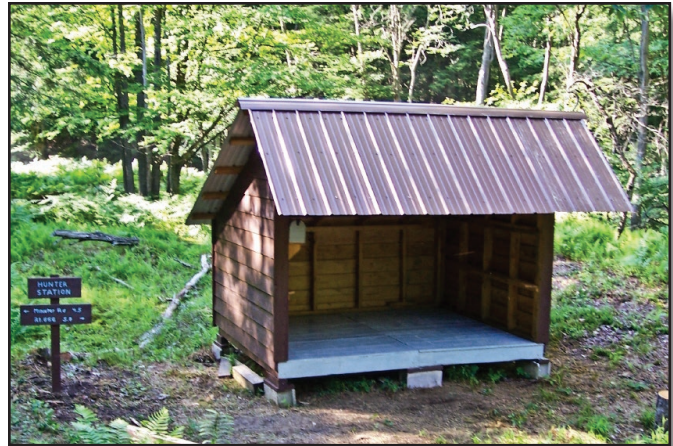
Figure 108—The entrance to the Hunter Station camp shelter at the Allegheny National Forest is raised above the ground.
