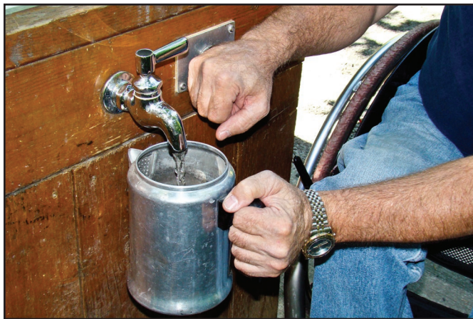
Figure 104—A solar pump provides pressure for this water spigot. A camper uses accessible controls to fill his coffee pot.
