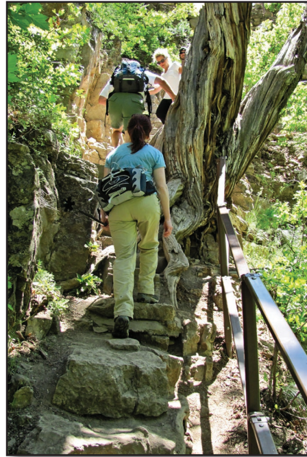
Figure 125—The combination of running slope and cross slope on the trail to Hanging Lake is so severe for such an extended distance that the entire trail was exempted from the technical requirements.
