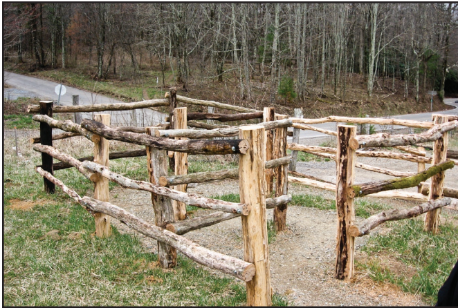
Figure 47—The winding configuration of this rustic chicane where the Appalachian Trail crosses Tennessee Highway 91 and the Osborne farm allows pedestrians to pass through the fence to use the trail but keeps motorized users out and horses inside the farm fence.
