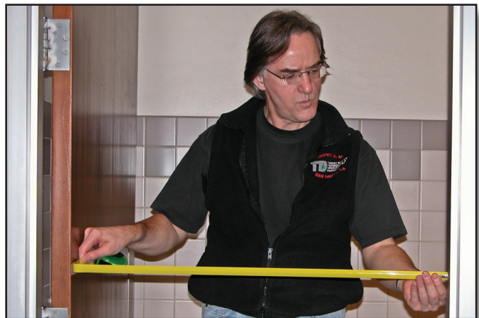
Figure 14—All doorways must have a minimum of 32 inches (815 millimeters) clear width.
