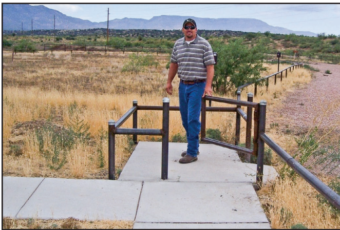
Figure 48—A steel kissing gate on the Prescott National Forest prevents passage by motor vehicles. The design balances the principles of the Built Environment Image Guide with the needs for access control. Sturdy, vandal-resistant materials were needed to discourage determined off-road vehicle users.
