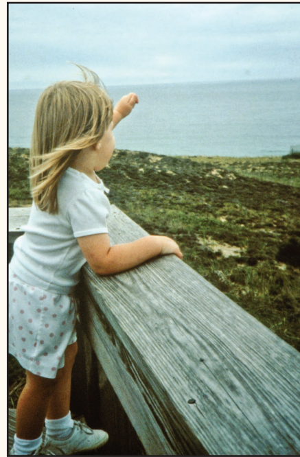
Figure 67—Caution: Railings with horizontal rails make an inviting ladder for small children.
