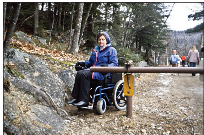
Figure 21—This road closure gate does not provide enough clearance to allow pedestrian passage.
